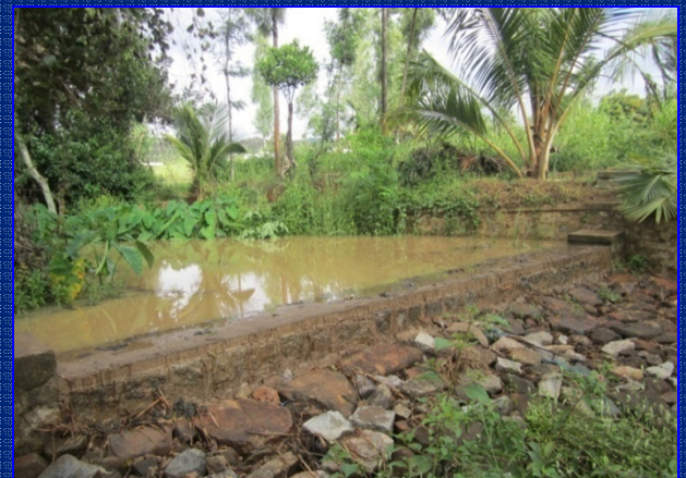
Heightening of check dams
