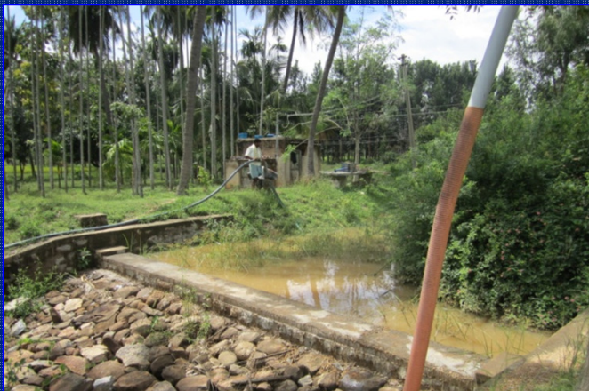
Heightening of check dams
